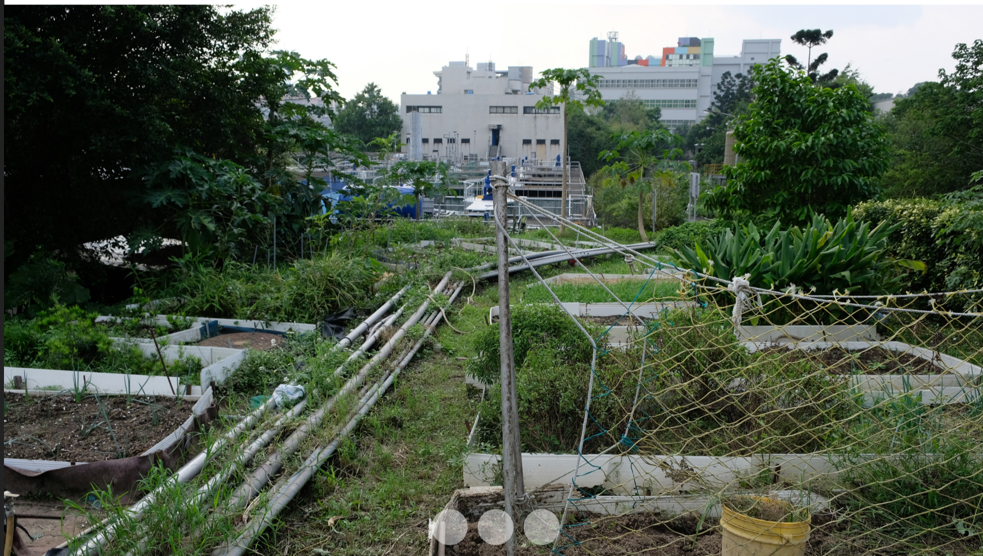
Outside the plant: wastewater recycling facility and community garden.
